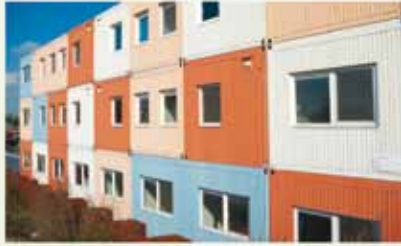
Figure A. These student apartments were made from recycled steel shipping containers. (Hansenn/Shutterstock.com)
